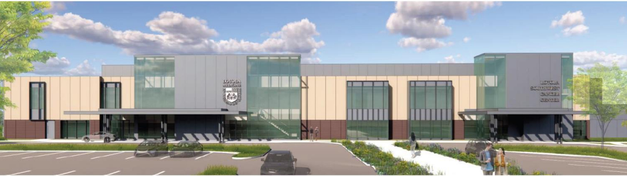
Second Proposal Option 1 - incorporated a brick base around the building. This image provides 5% face brick; 34% precast panels; 31% glass and 29% metal panels
